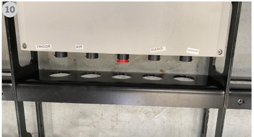
13. Mount the solenoid block in position.
